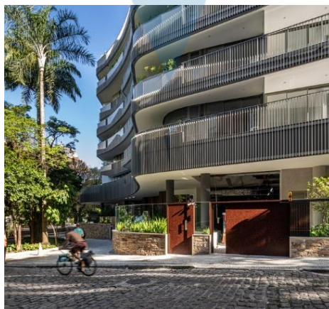
Gambar 2.16 Ruang Sosial di Depan Brisa Apartments Sumber: Archdaily
