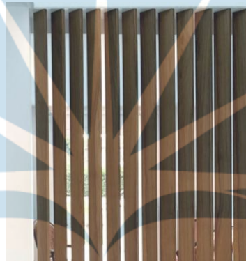
Gambar 5. 19 Perforated Wall Balkon Unit Apartemen
