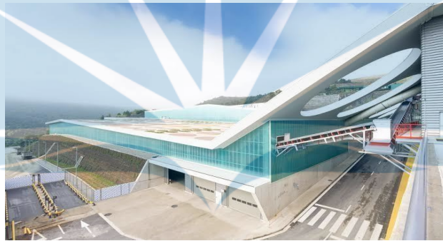
Gambar 2.26 : Waste Treatment Facility (Barcelona)
