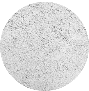
DINDING FINISHING BETON
