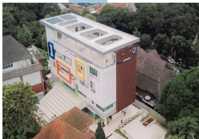
Gambar 2. 18 Gedung ITB Innovation Park Sumber : ITB Innovation Park
