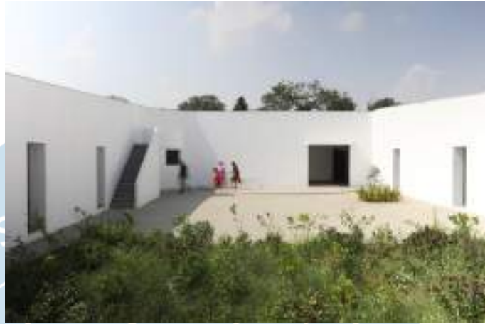
Gambar 2.1 School for Blind and Visually Impaired Children
