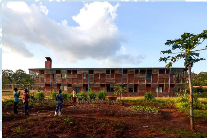
Gambar 2. 16. Fasad Children's House Busajo Campus Sumber: Pietro Savorelli
