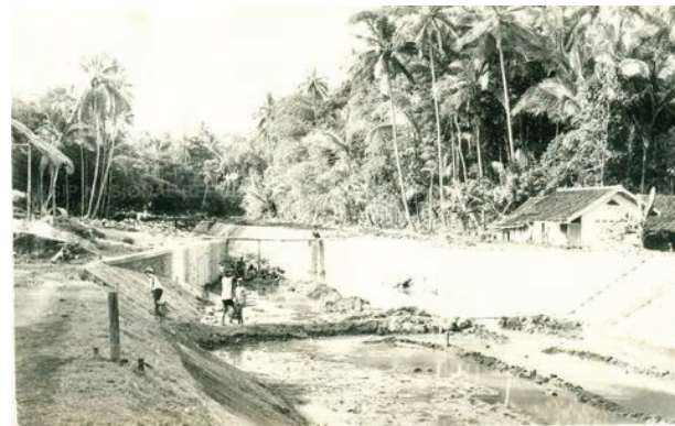
Fig.2. Left: Excavation work for the Walet drainage channel, Phase II of the Mataram Canal rainwater drainage excavation. Right: Phase I construction of the tertiary Mataram Canal, quarter-channel system. Source: National Archives of the Republic of Indonesia ( https://mowid.anri.go.id/index.php/fdpa-028-1-2 ) accessed on Friday, 21 March 2025.
