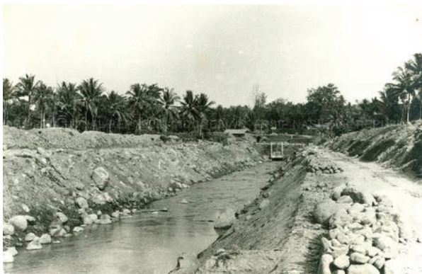
Fig.2. Left: Excavation work for the Walet drainage channel, Phase II of the Mataram Canal rainwater drainage excavation. Right: Phase I construction of the tertiary Mataram Canal, quarter-channel system. Source: National Archives of the Republic of Indonesia ( https://mowid.anri.go.id/index.php/fdpa-028-1-2 ) accessed on Friday, 21 March 2025.
