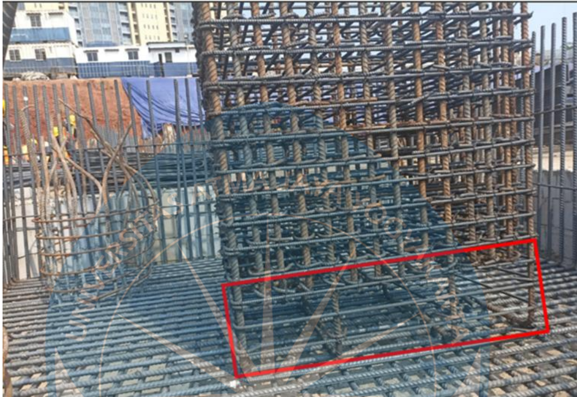
Figure 2. 15. Column Connection Method to Pile Cap
