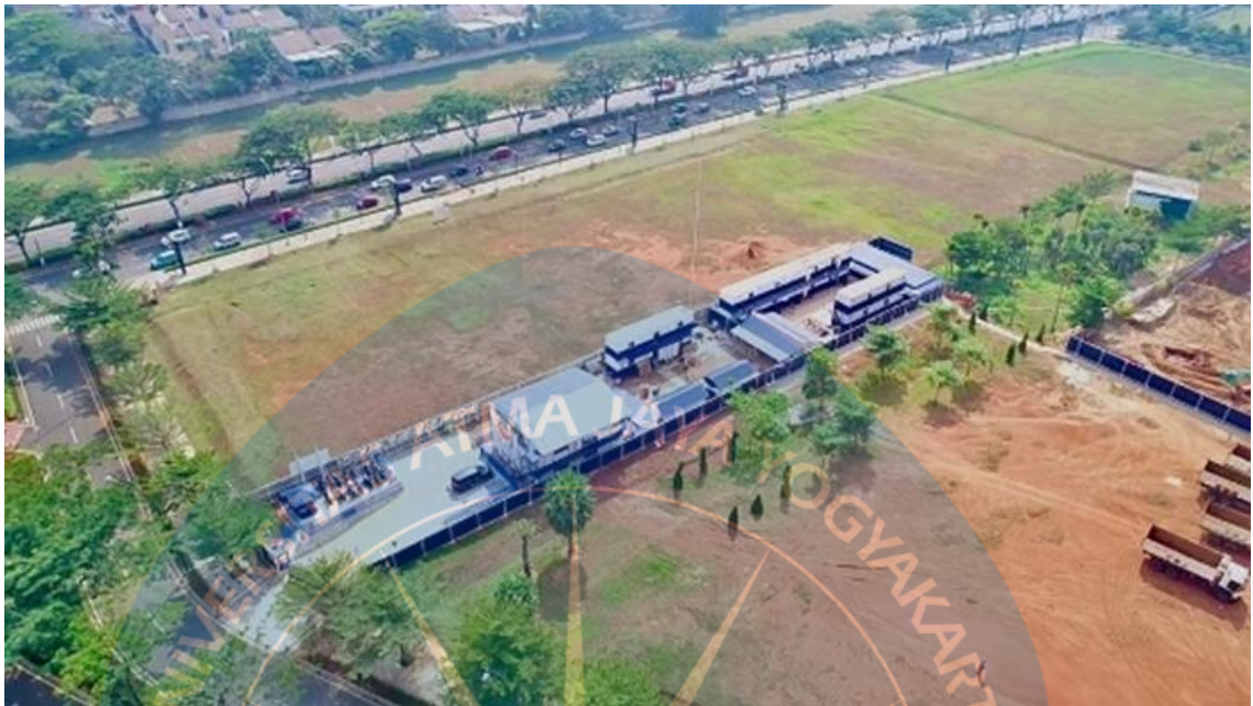
Figure 2. 2. Site Office of Novotel Hotel Project
