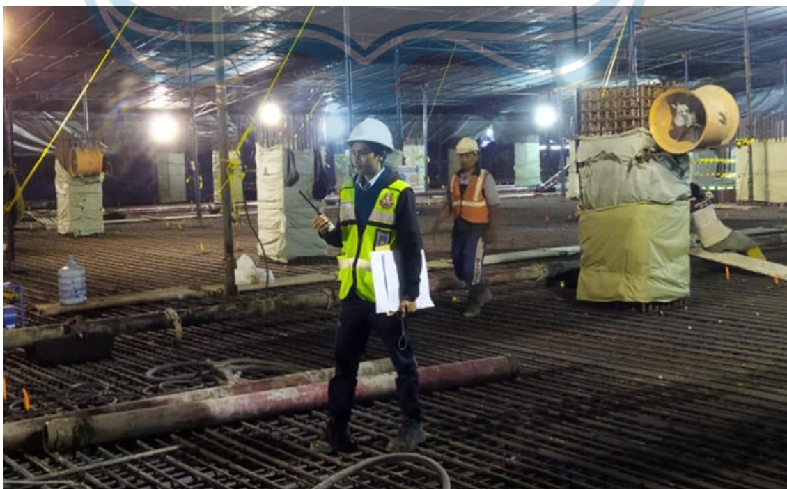
Figure 2. 35. Lower Concrete Pump Post
