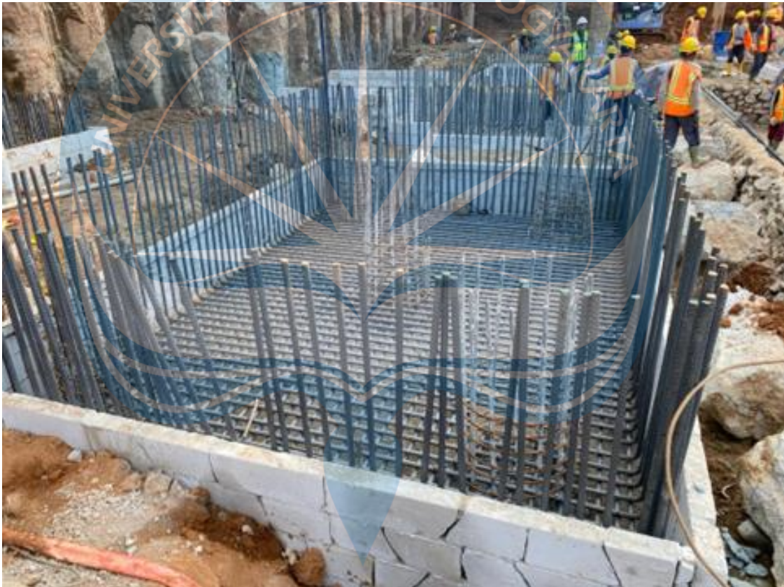
Figure 2. 6. Pile Cap Reinforcement Work
