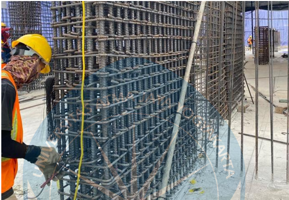
Figure 2. 13. Shear Wall Reinforcement Work
