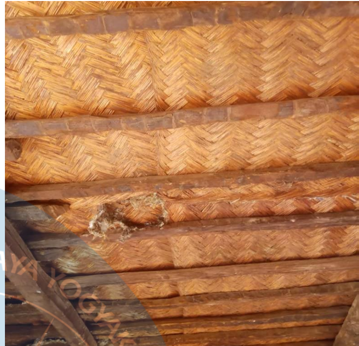
Thresh ceiling of a Lagos traditional mud house
