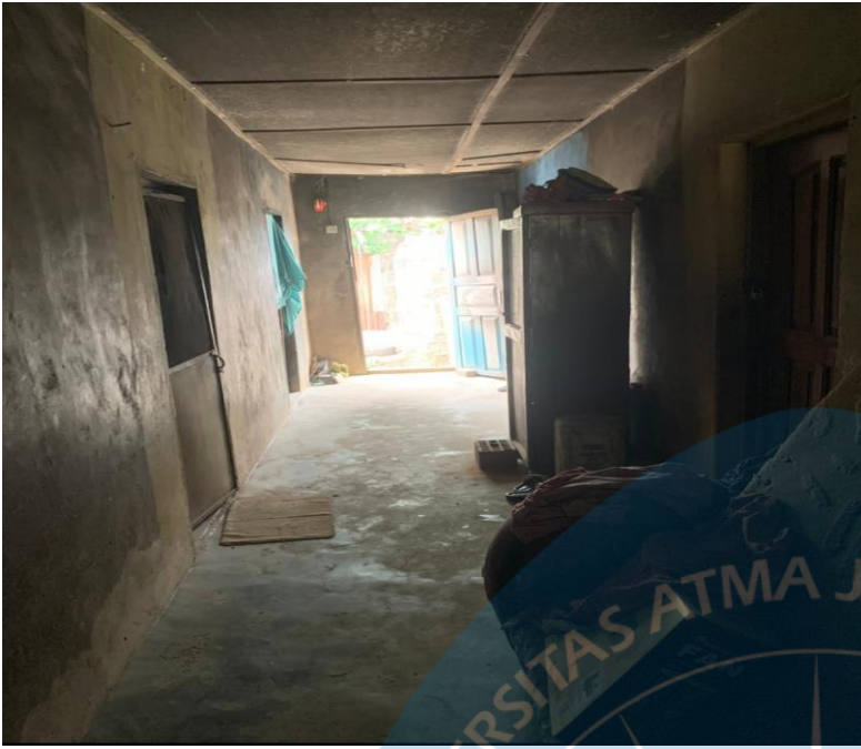
Central Hallway that leads to all other spaces
