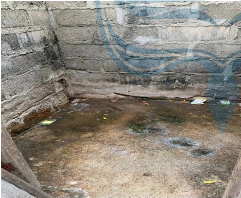
bBathroom, usually located outside of the house
