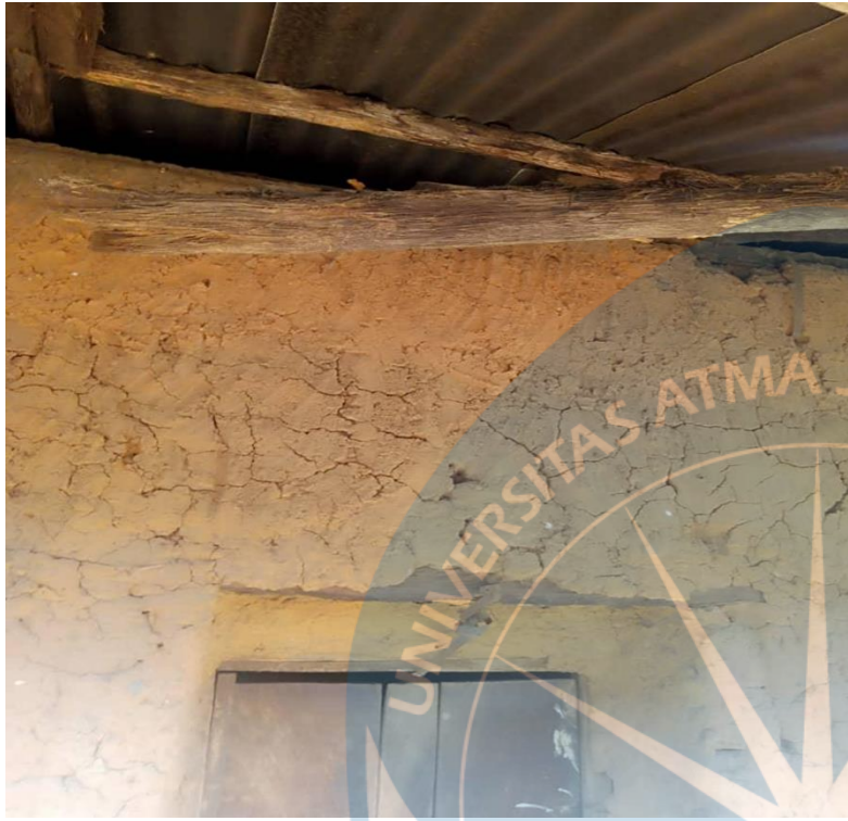
Traditional home in Lagos with mud brick walls with aluminum roof sheet
