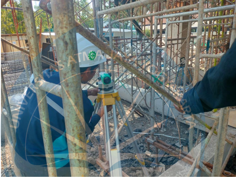
Gambar 2.1a Setting Alat Auto Level
