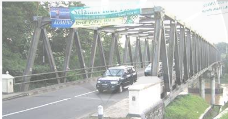
Gambar 2.2 Jembatan Rangka / Truss Bridge (wiryanto.wordpress.com 2008)
