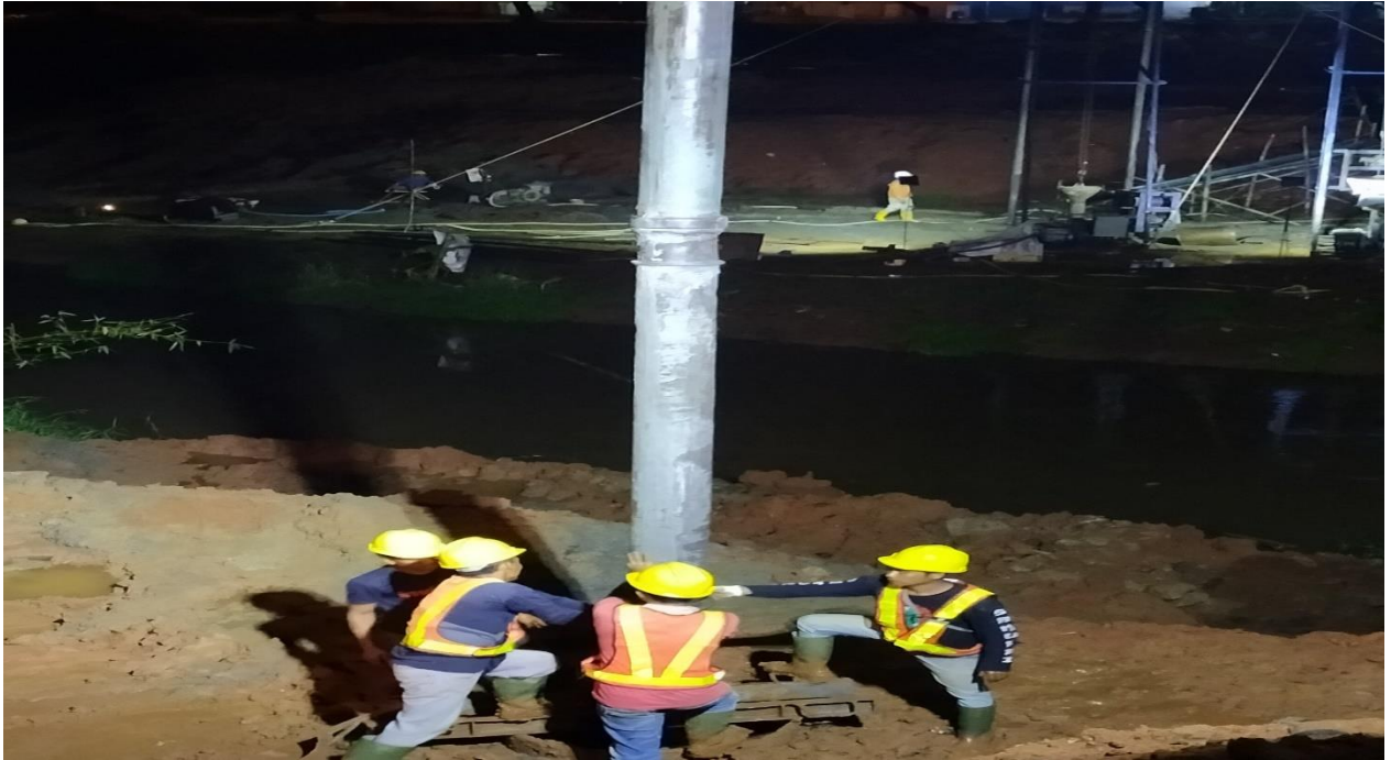
Instal pipa tremie
