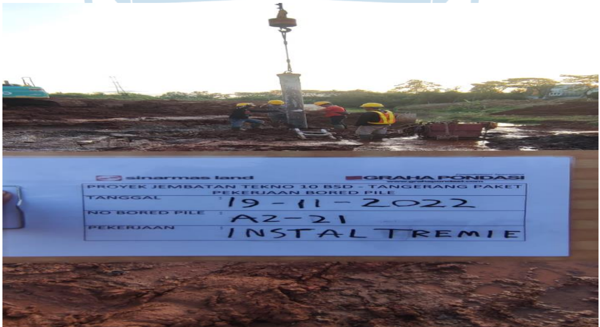
Dokumentasi monitoring instal pipa tremie
