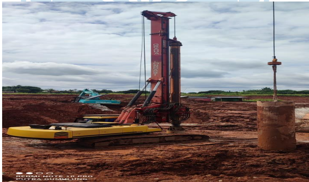
Proses instal casing kedalam lubang
