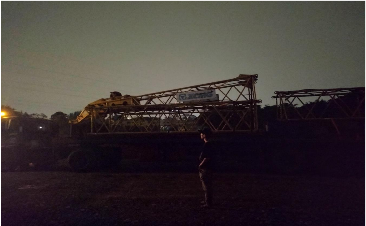
Mobilisasi Unit crane service
