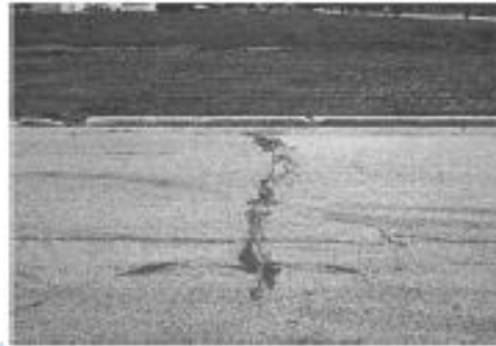
Gambar 3.4 (1) Low ; (2) Medium ; (3) High Longitudinal & Transversal Cracks
